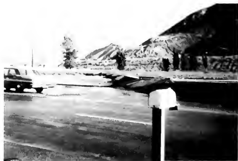
Photo 1. Frontal fault scarp of the Tujunga fault segment on Foothill Boulevard just west of the Foothill Nursing Home, which has since been razed (locality 90, plate 3). Note water in street from ruptured water mains. Photo taken by F. Harold Weber, Jr., at 9:00 a.m., February 9, 1971.
